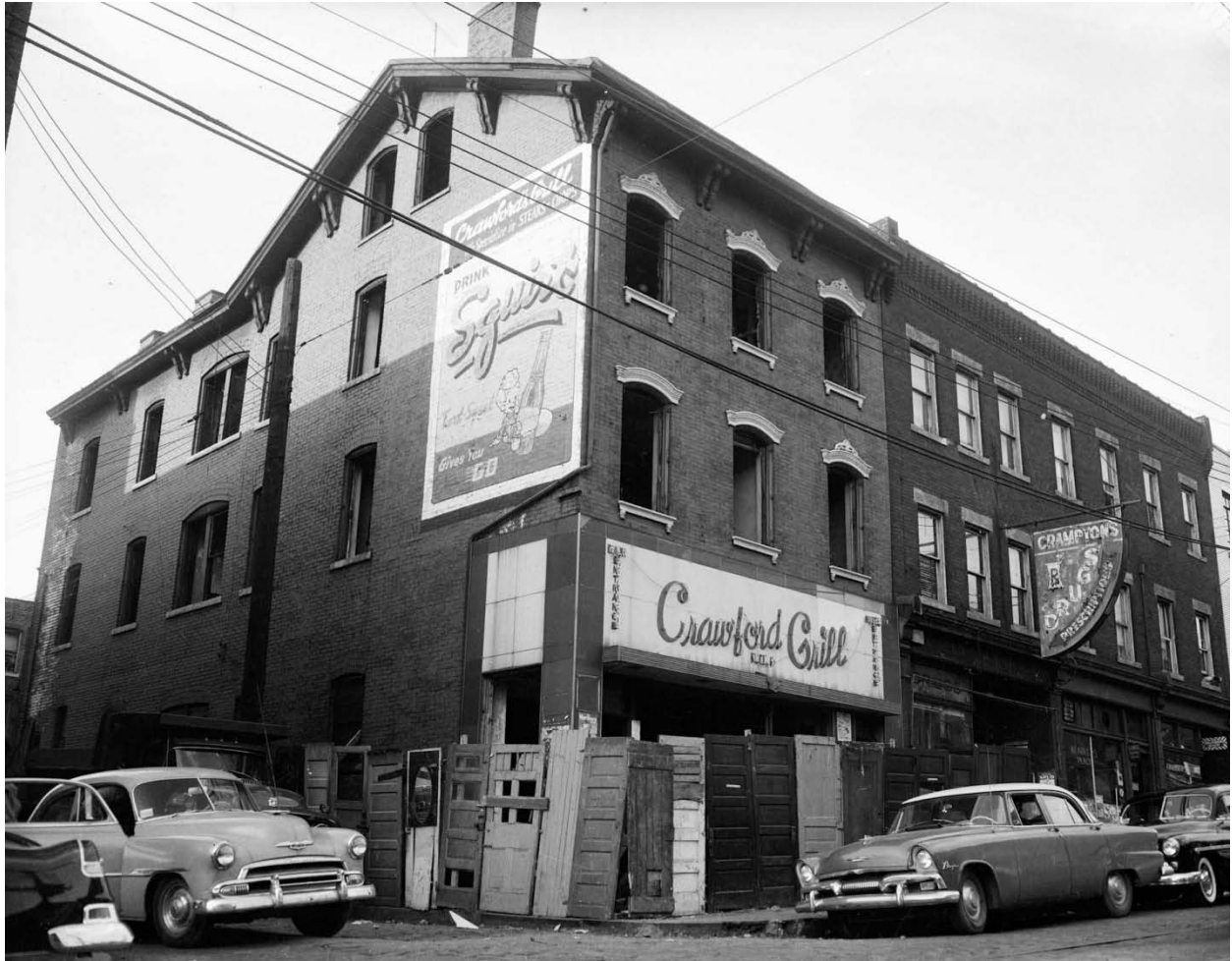
Figure 13 The Crawford Grill, boarded up after it was gutted by a fire, 1956 (Charles “Teenie” Harris, Carnegie Museum of Art, Pittsburgh: Heinz Family Fund, 2001.35.2363)
